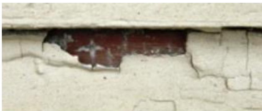
Brookfield Depot peeling paint. ©2012 Ted Schaar
